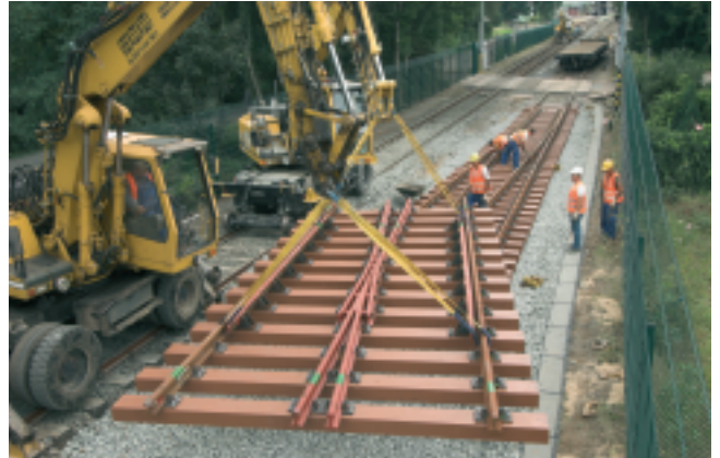
Installation of Turnout at Bayer Leverkusen Plant
