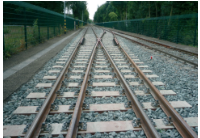
Final Installation of Turnout
